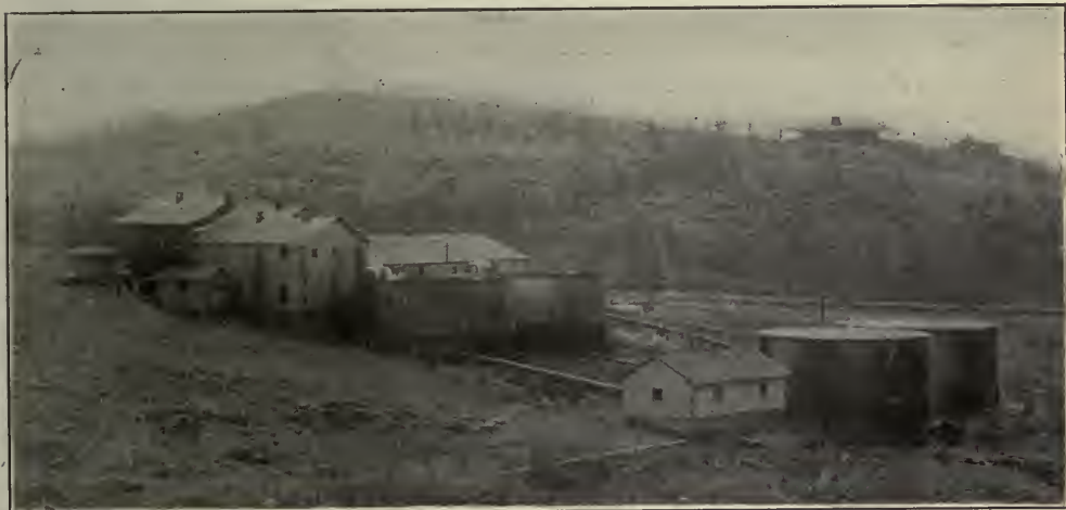
THE LAWTON, OKLA., FILTER PLANT AND STORAGE TANKS
